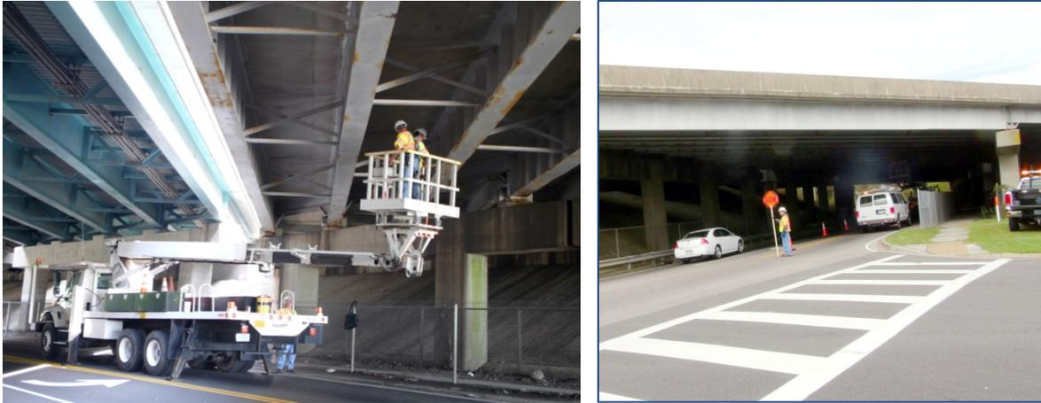
Figure 6: Installation of AE transducers on the bridge structure.
